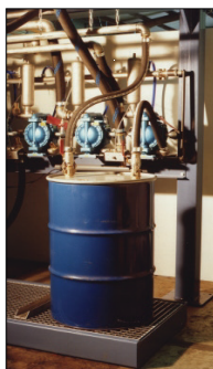
Dispensing directly out of drums.
